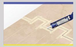
Using gentle pressure, carefully apply the Micro Joint material into the open grout line. (You may find it convenient to apply masking tape to the sides of the grout line if unsure of accuracy). Ensure the Micro Joint material is filled level to the surrounding grout level. Check and top up if the level drops.
